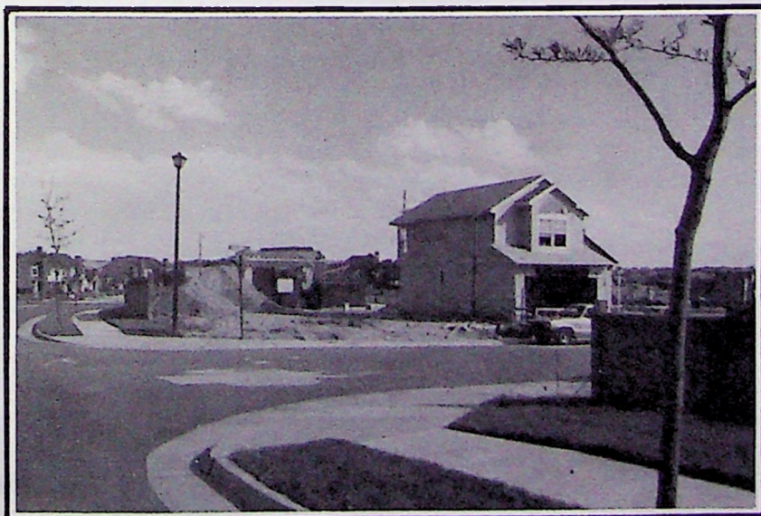
New home under construction southeast of Aurora, CO. Several subdivisions are planned for this area in the next five years.
