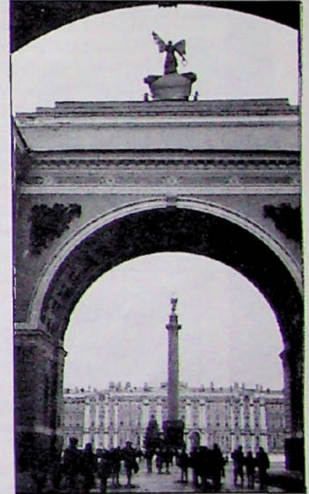
Arches leading into courtyard in front of the Hermitage (St. Petersburg)
