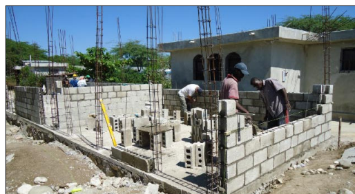
Building the block walls
