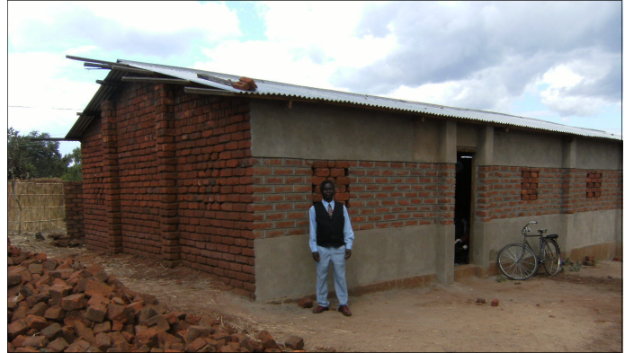
An example of a church that has been built with tin roof and improved mud bricks.
