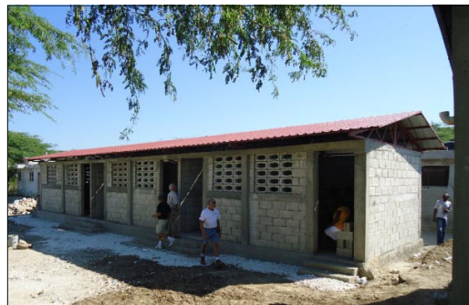
The nearly finished building
