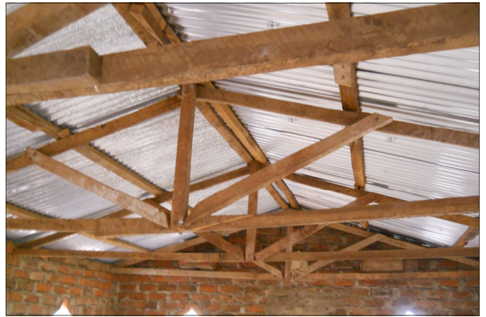
Masenjelo Church—rafters and roof
