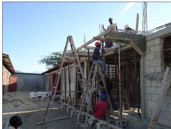
First floor construction is nearly complete
