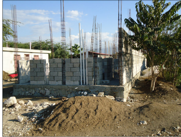
Construction of first story floor and walls
