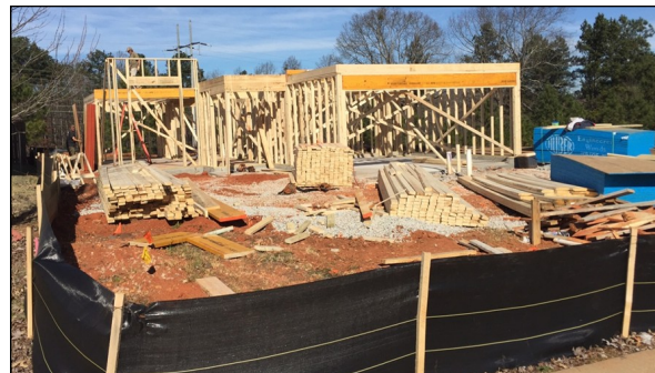
New student housing construction
