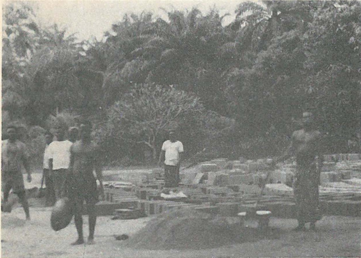
Nigerians making blocks for an additional building for their school.
