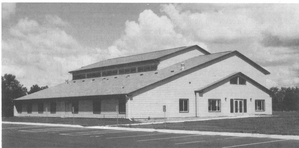
The completed Pine Grove Bible Church at Minneapolis, Minnesota.
